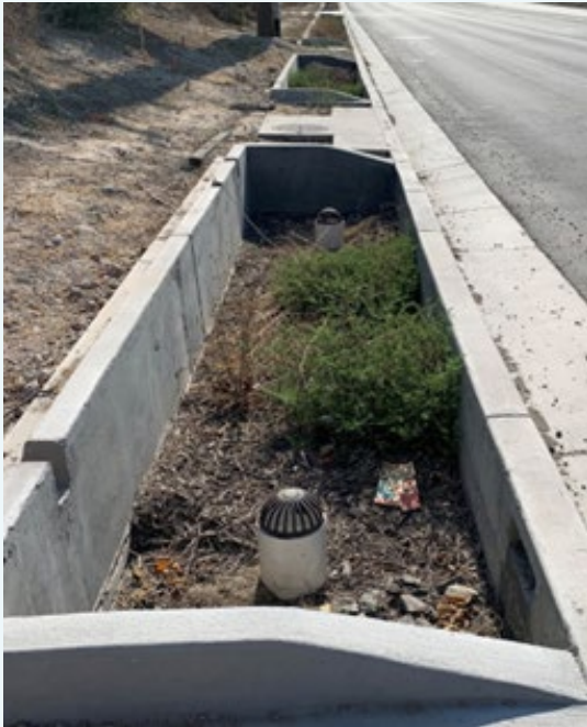
Hydromodification biofilter located along a roadway to filter and intervene with contaminants in stormwater runoff, including microplastics and vehicle tire wear. Photo credit: SCCWRP.
