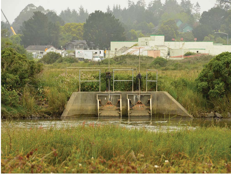
Figure 9. Existing dike and tide gates on right bank of Elk River in Area 1, that will be removed.
