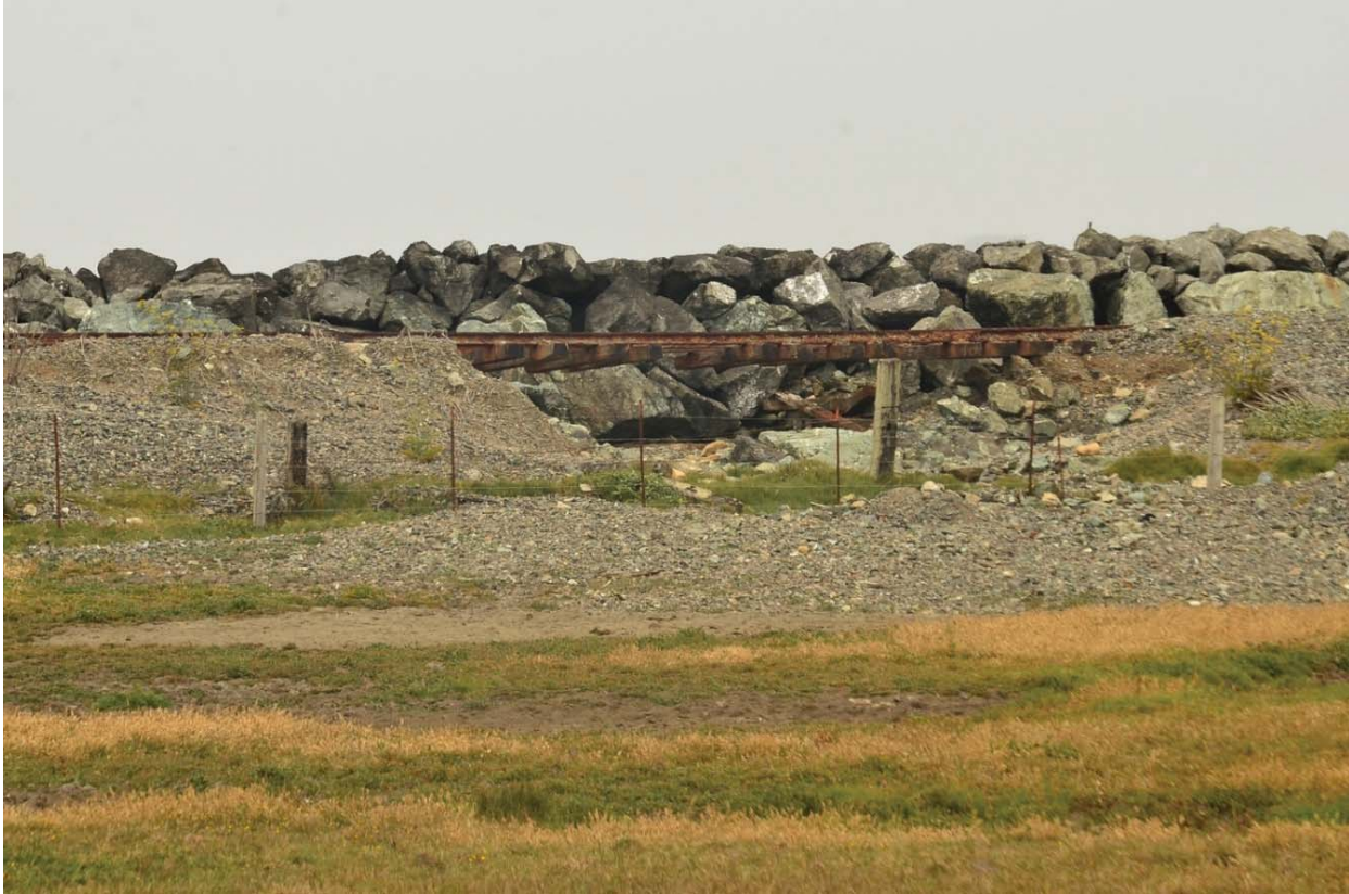
Figure 27. The existing railroad grade after the 2015-2016 king tides and storm surge erosion, showing fill of Area 2 wetlands.
