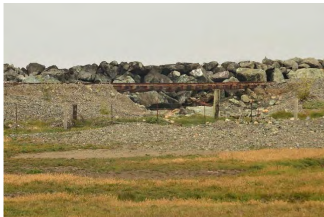
Looking west at the existing railroad grade adjacent to Area 2 after the 2015-2016 king tides and storm surge erosion, showing washout of ballast into Area 2. A tidal ridge will be constructed along the railroad grade, preventing further washout of ballast into the area to be restored to marsh.
