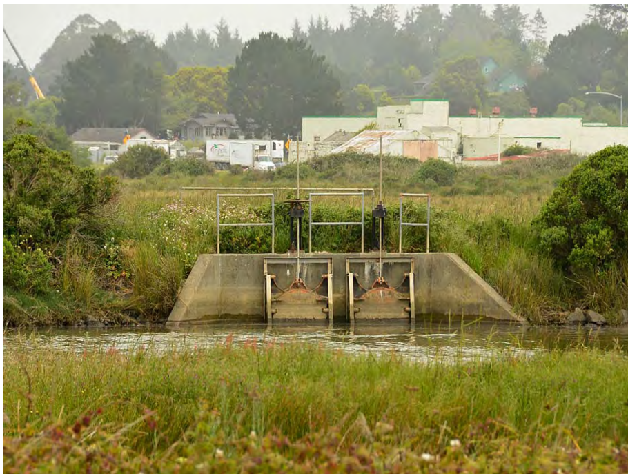
Existing dike and tide gates on right bank of Elk River in Area 1. This tidegate will be removed.
