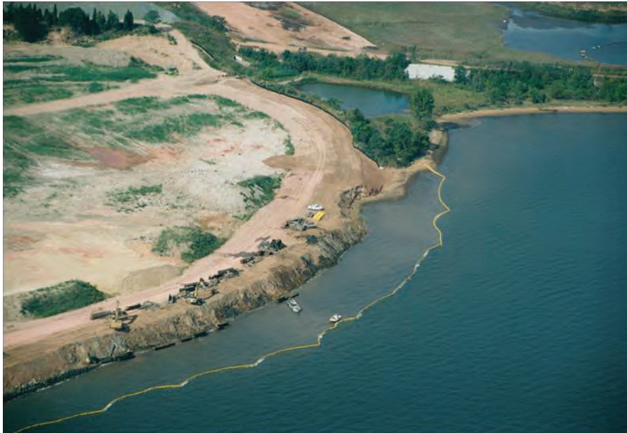
Photo A. Turbidity control with containment fencing
