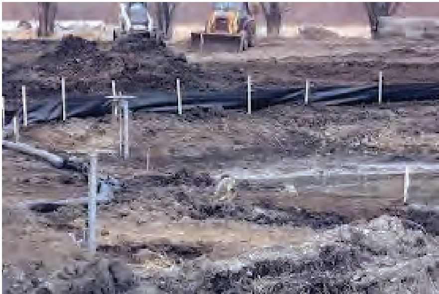
Photo C. Silt Fencing around a channel
