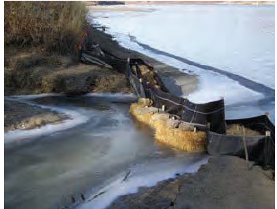
Photo B. Turbidity control with containment fencing www.terraerosion.com
