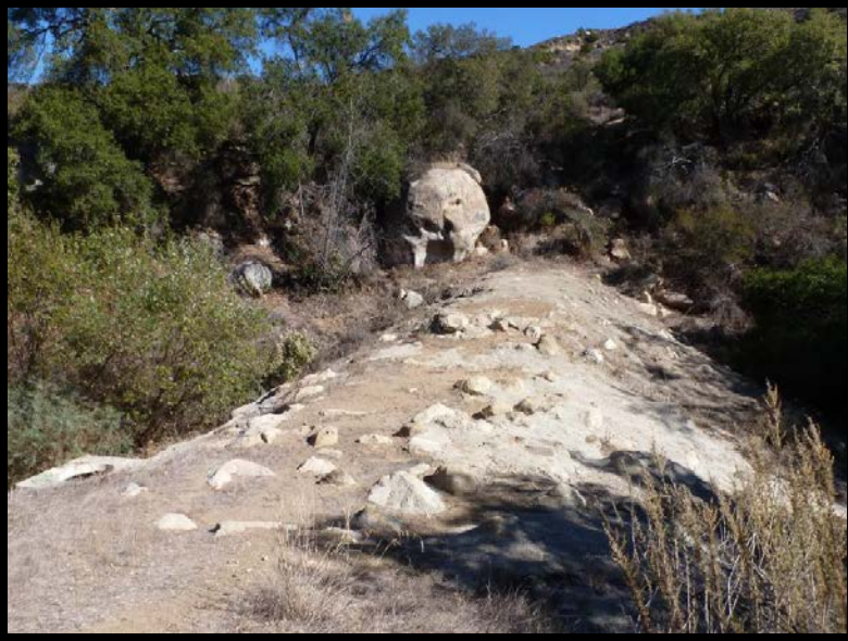
Rattlesnake Creek Debris Basin: Grouted Rock Dam
