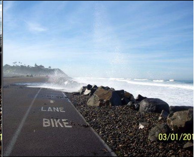
Flooding of HWY 101
