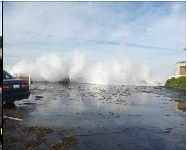
Wave Attack on Revetment Fronting Restaurant Row
