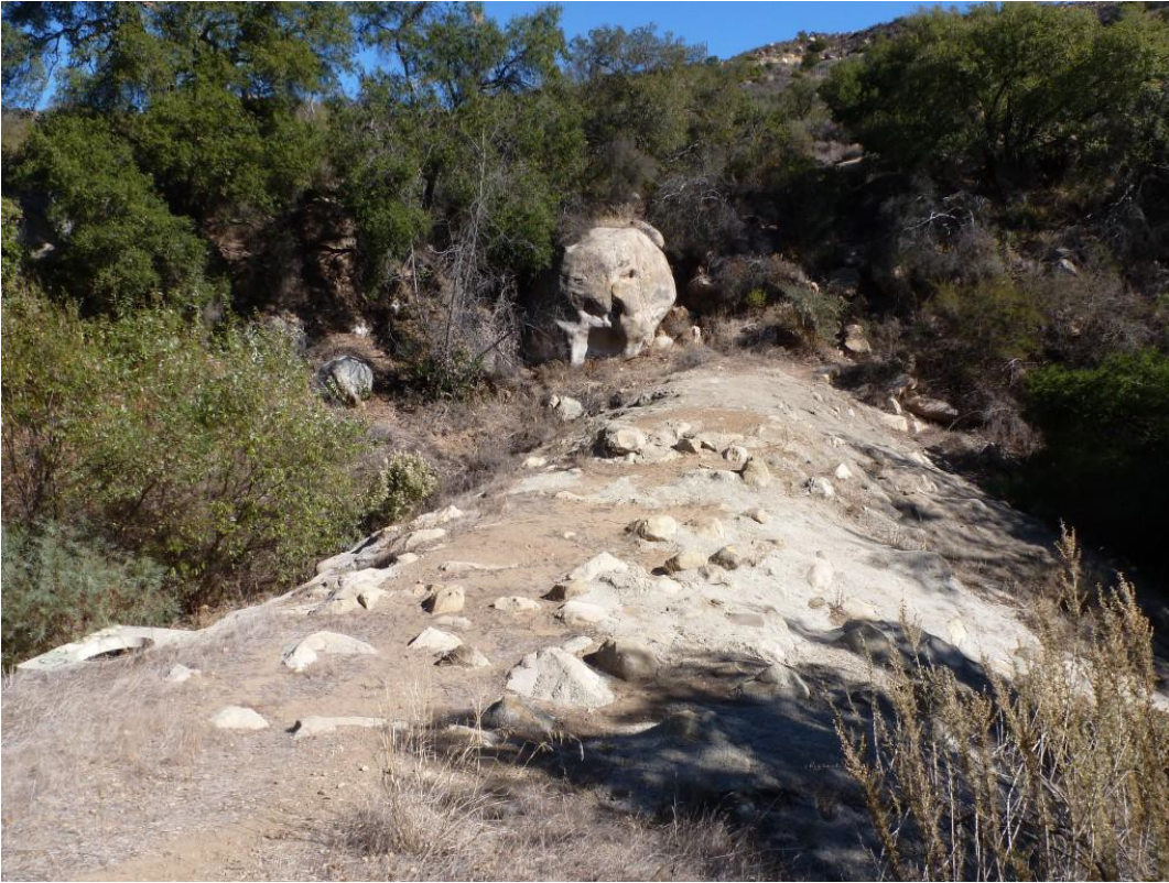
Figure 1: Rattlesnake Creek Debris Basin - grouted rock dam - facing east
