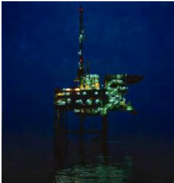
Fig. 4. Off shore platform equipped with low-red exterior lighting.
